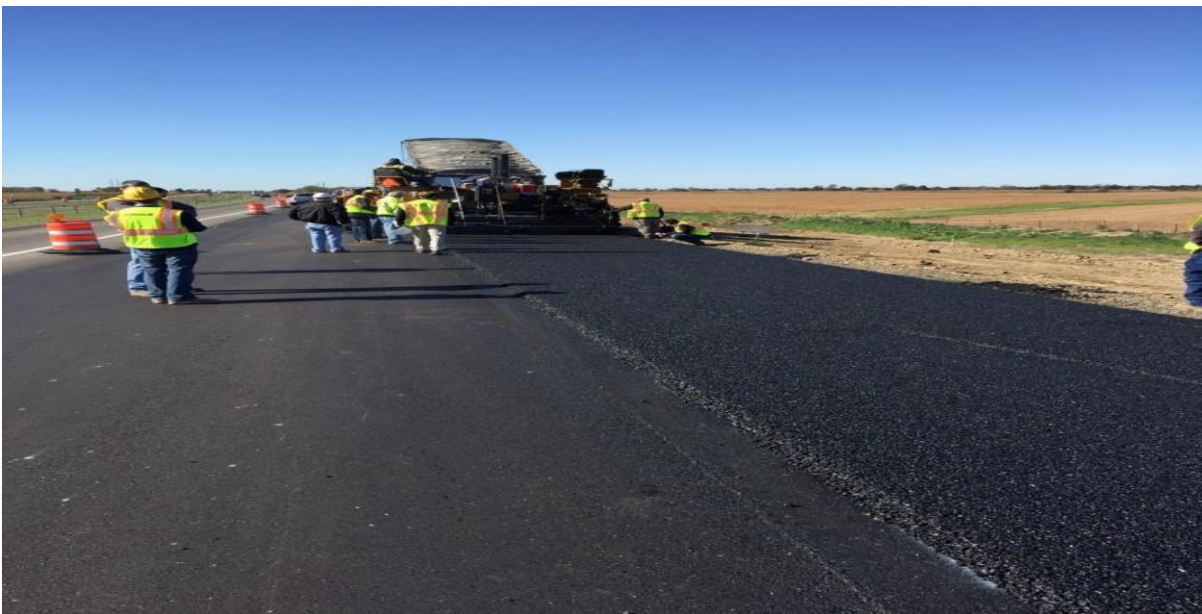
Figure 52 Rubberized Asphalt Concrete
