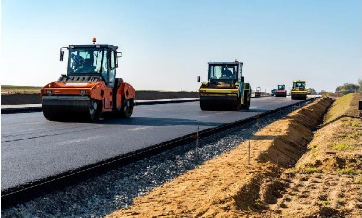
Figure 4 Construction of Typical Flexible pavement Roadway
