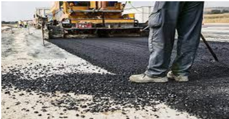
Figure 42 Sand- Asphalt Mix Application
