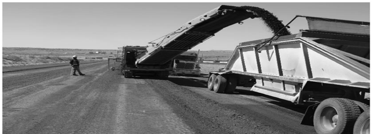
Figure 50 Milling of Reclaimed Asphalt Surface
