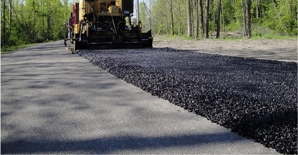
Figure 46 Cold Mix Asphalt Application
